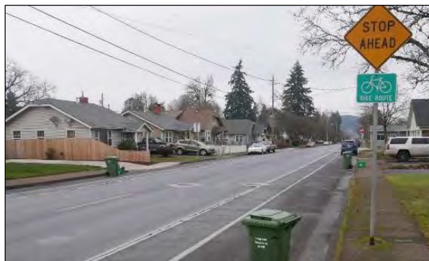
Figure 3-13. Typical Striped Bike Lane and Supplemental Signage
