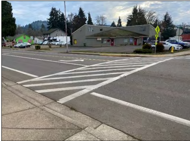
Figure 3-26. Marked Crosswalk with RRFB and Median Refuge on Row River Road
