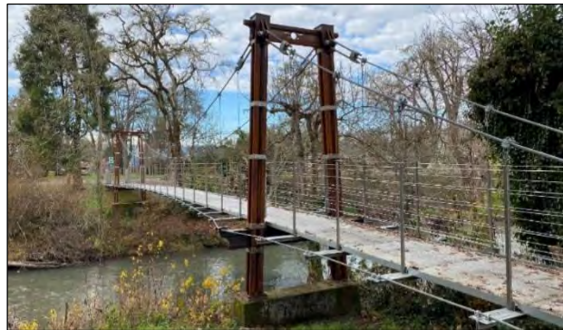
Figure 3-12. Swinging Bridge at Madison Avenue
