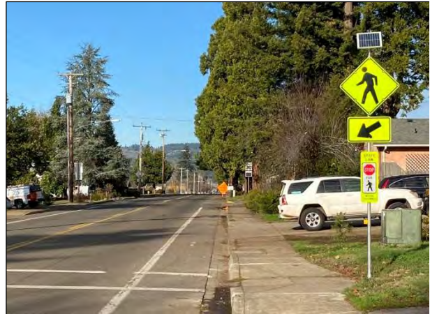
Figure 3-26. Marked Crosswalk with RRFB and Median Refuge on Row River Road
