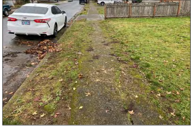
Figure 3-7. Example of Excessive Weed Growth on a Local Sidewalk
