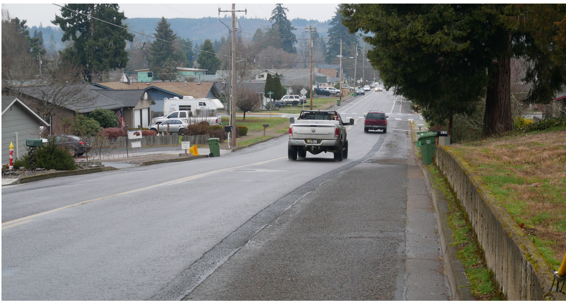
Sidewalk Gap on 6th Street
