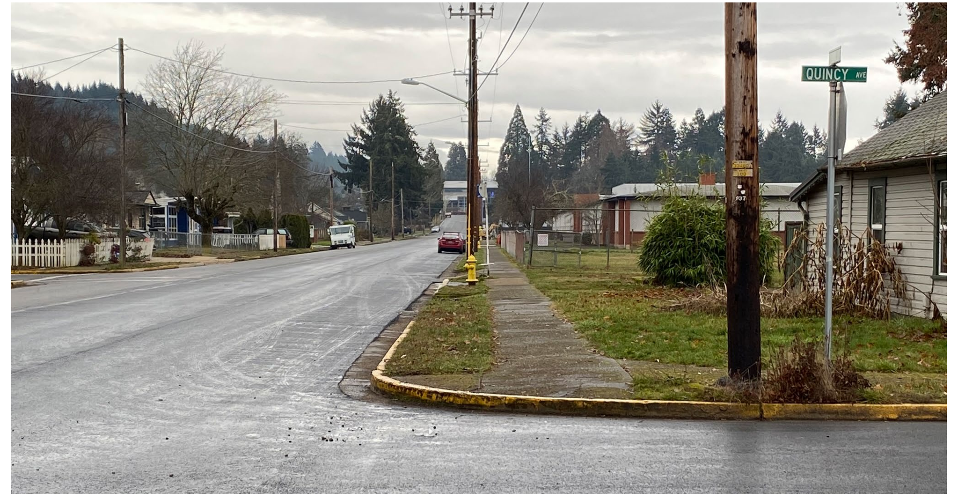
Missing Curb Ramps along Quincy Avenue
