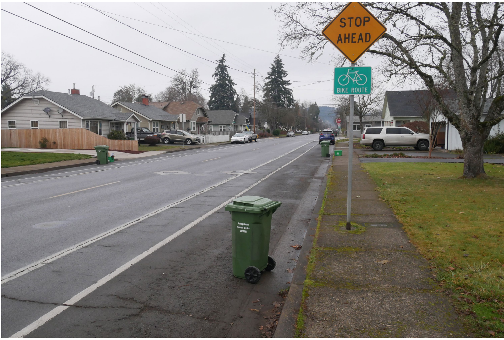
Typical Striped Bike Lane and Supplemental Signage
