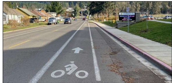
Figure 2-11. Typical Conventional Bike Lane
