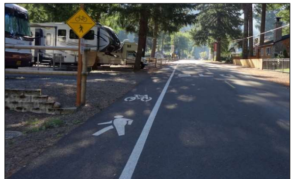
Figure 2-2. Typical Pedestrian Lane
