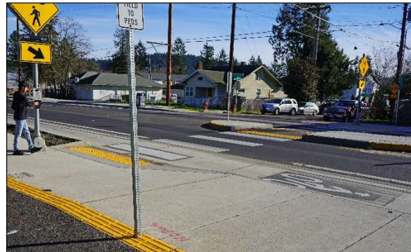
Figure 2-5. Typical Enhanced Crossing with Median
