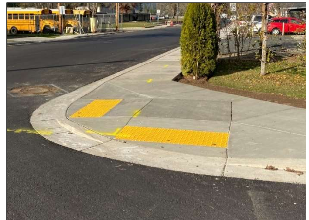
Figure 3-9. Recently Upgrade Curb Ramps near Lincoln Middle School
