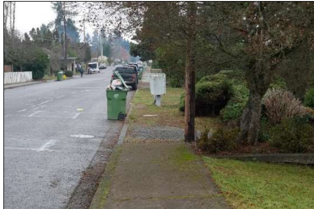
Figure 3-2. Intermittent Sidewalk Gap
