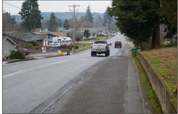
Figure 3-5. Sidewalk Gap on 6th Street
