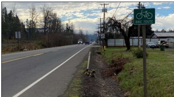
Figure 3-15. Rural Shoulder Bikeway on Highway 99 in Southern Cottage Grove
