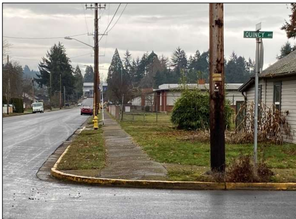
Figure 3-8. Missing Curb Ramps along Quincy Avenue
